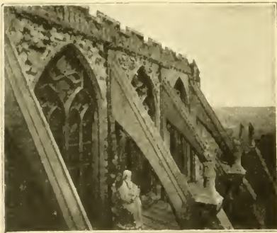
FLYING BUTTRESSES from the upper wall of Norwich Cathedral.
